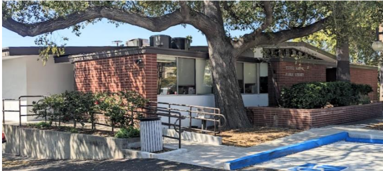
Northern/Entrance Façade, general view
