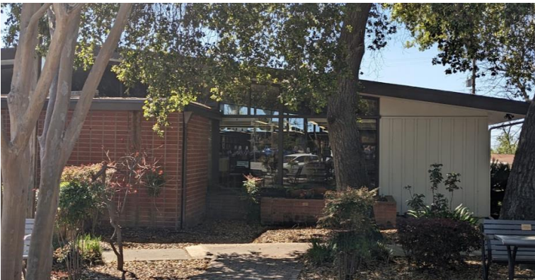
Northern/Entrance Façade, right side
