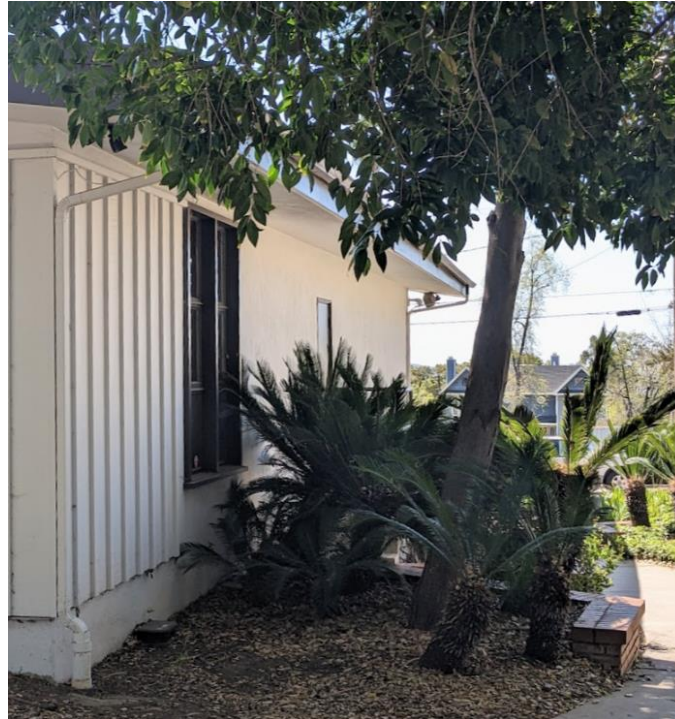
Western Façade, general view
