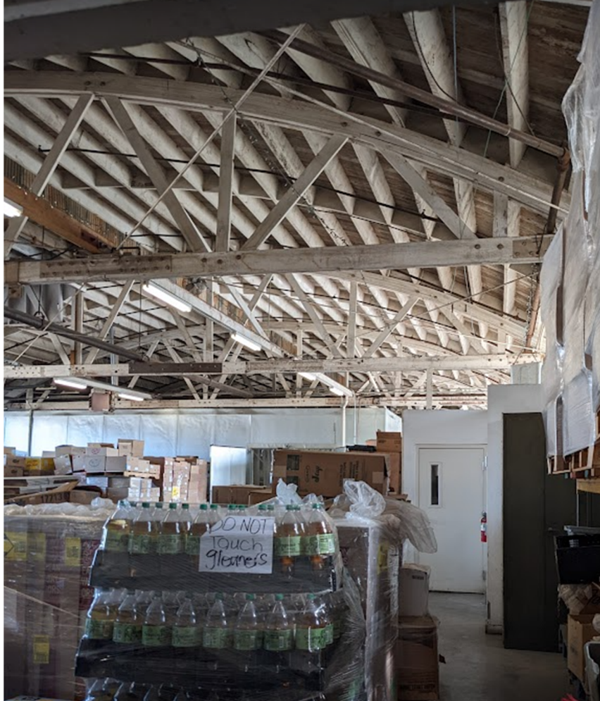
Second warehouse interior, looking east
