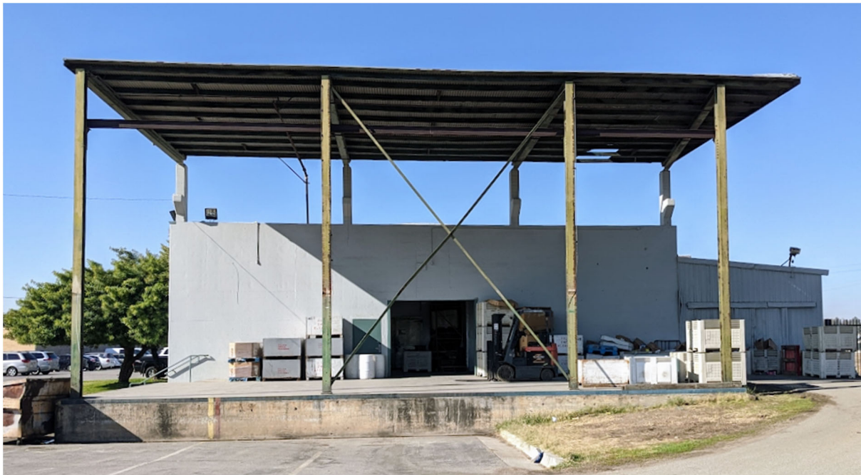
East façade (loading dock)
