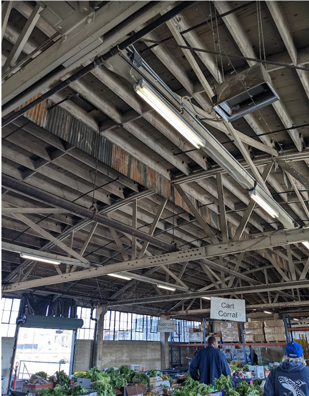
First warehouse interior, looking northeast
