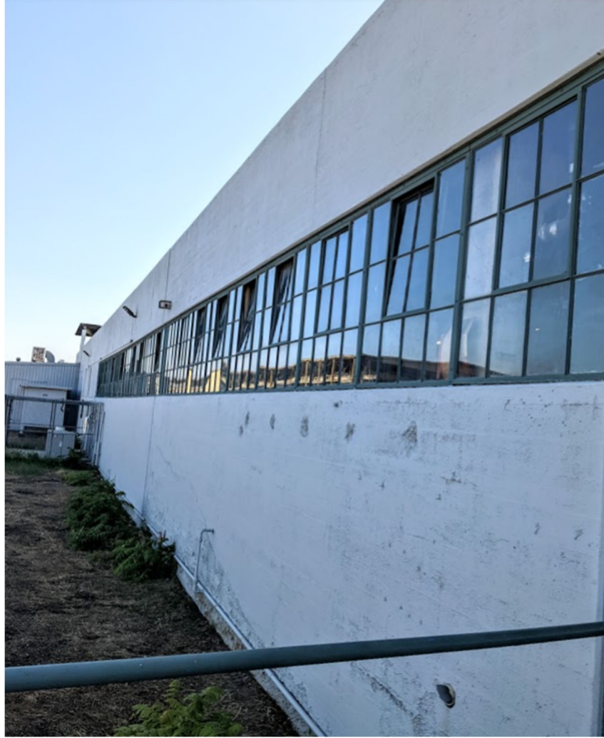
North façade, looking east from porch
