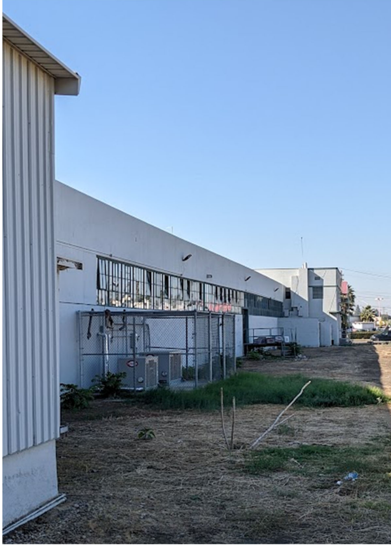
North façade, view looking southwest
