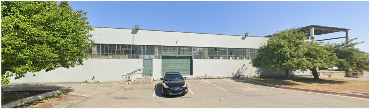
South façade, left portion
