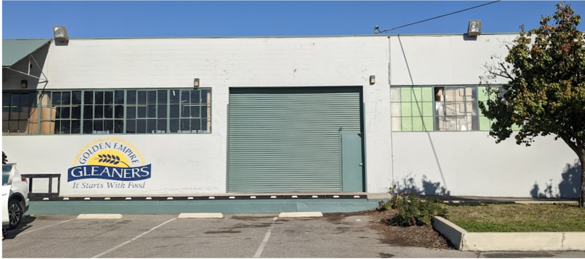
South façade, central portion
