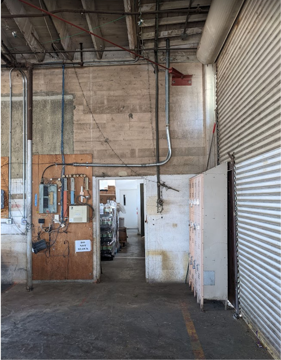
Partition wall between first and second warehouse spaces (looking east)
