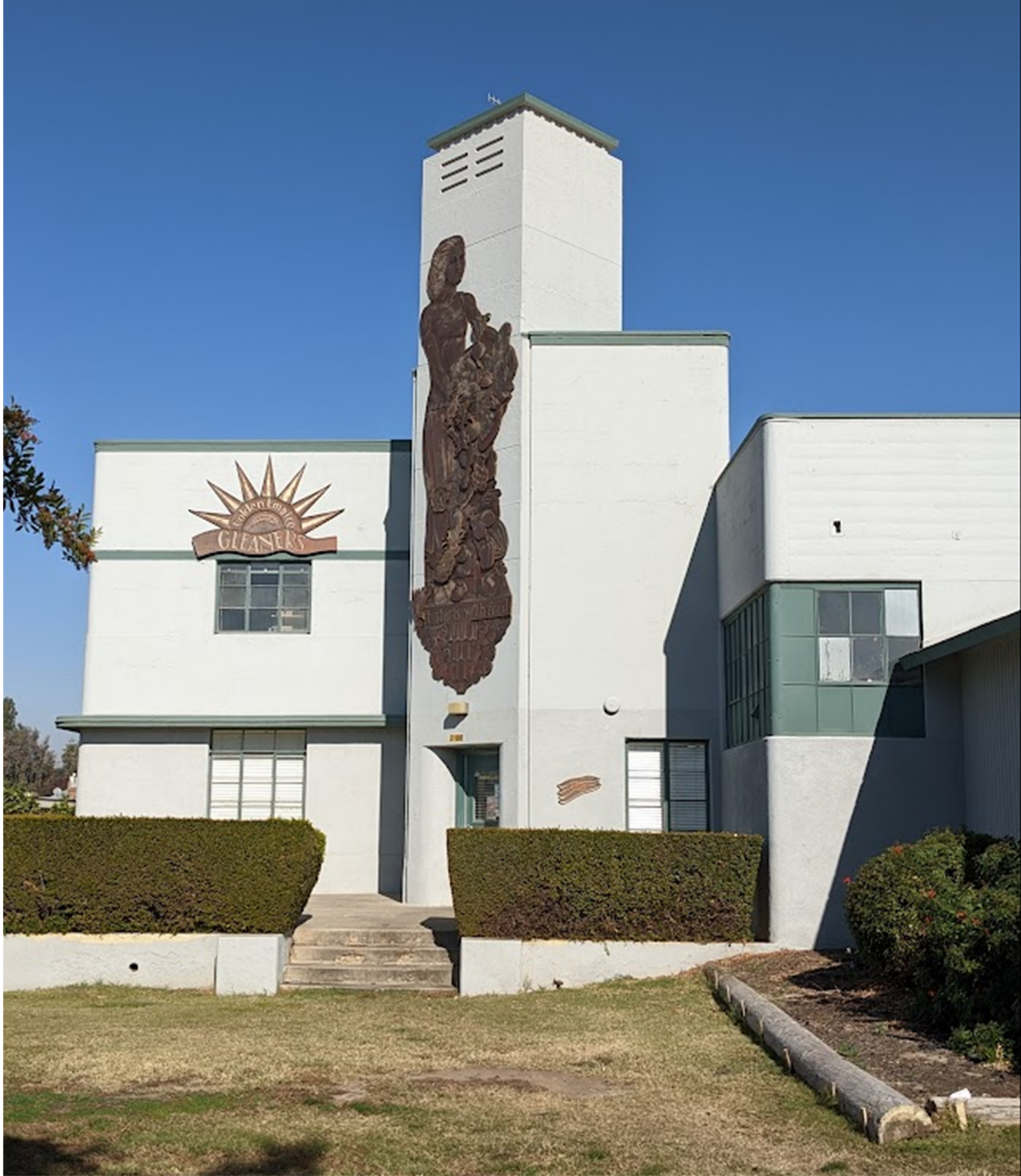
Office block entrance, looking northeast
