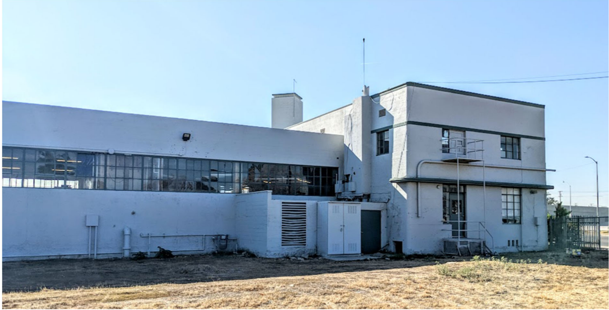
North façade, right portion
