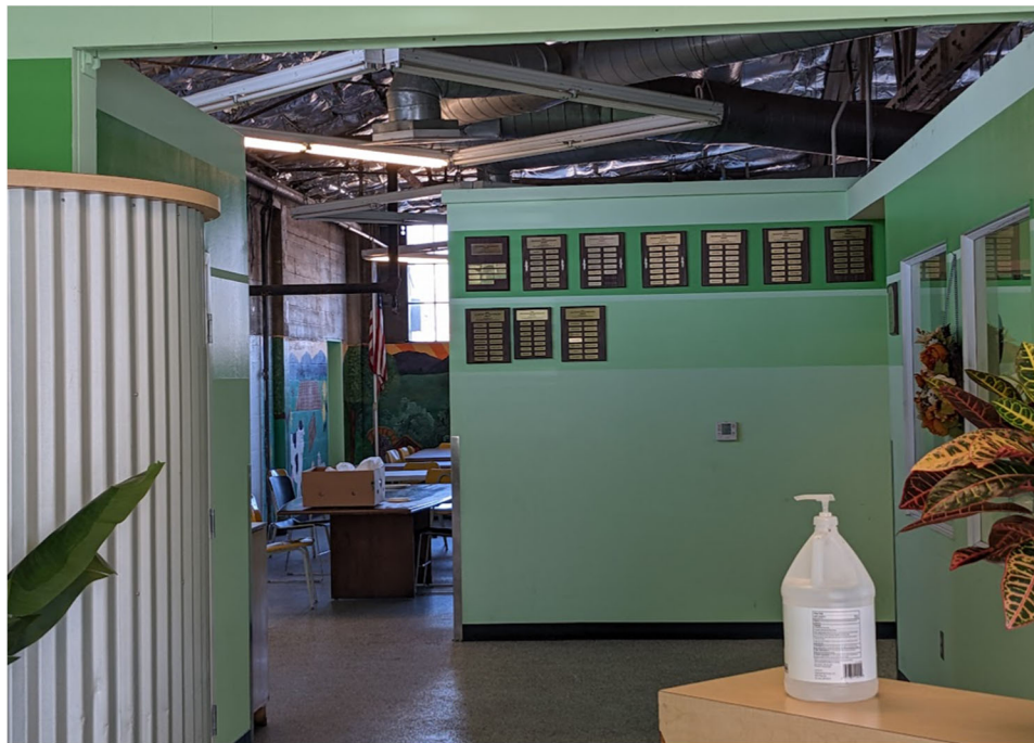
First floor of office block, looking west
