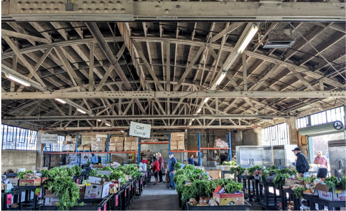
First warehouse interior, looking east
