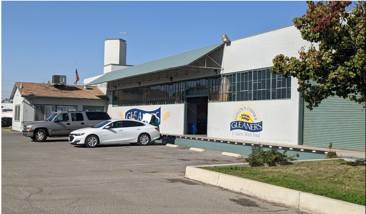
South façade, looking west toward southwest addition and office tower
