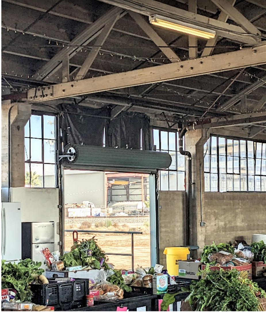
First warehouse interior, north wall showing roll-up door leading to porch
