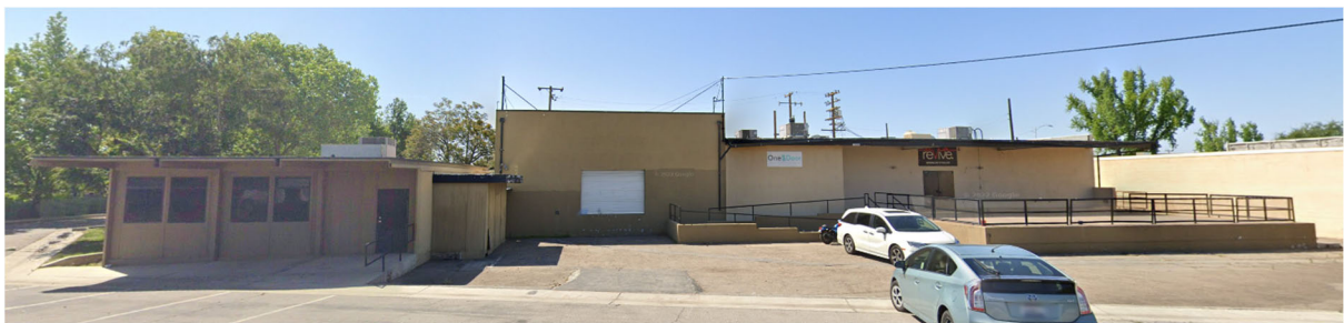
Central Kitchen (south outbuilding), north façade
