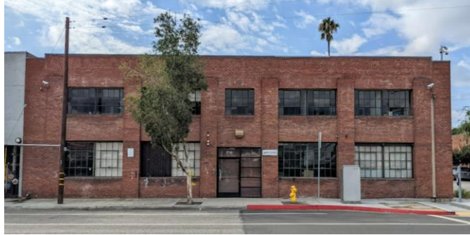
Figure 14. Primary/Northern Façade SOURCE: Sapphos Environmental, Inc., 2022
