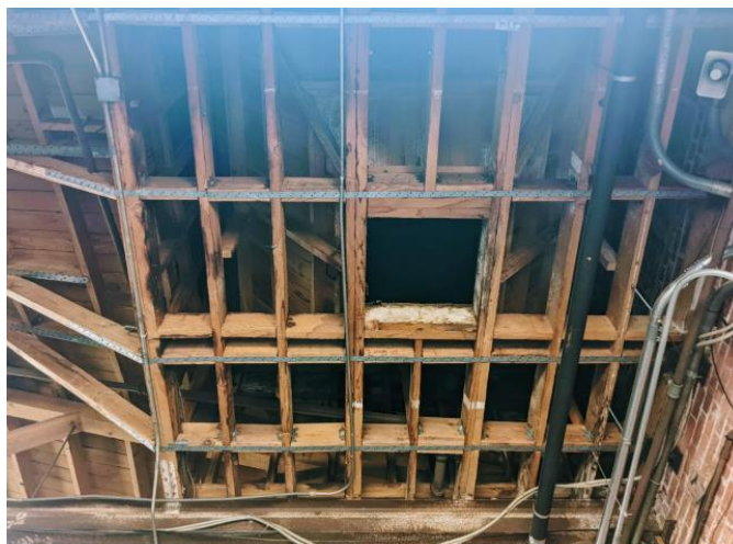
Figure 19. Exhaust Fan Aperture, Main Factory Space SOURCE: Sapphos Environmental, Inc., 2022
