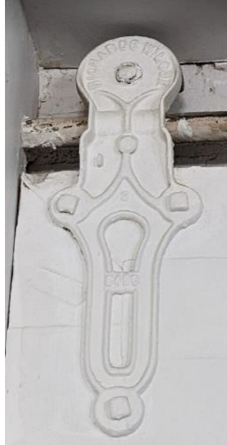
Figure 28. Closeup of Richard-Wilcox 542C Roller SOURCE: Sapphos Environmental, Inc., 2022
