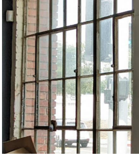
Figure 24. Mid-Sash Pivot Windows SOURCE: Sapphos Environmental, Inc., 2022
