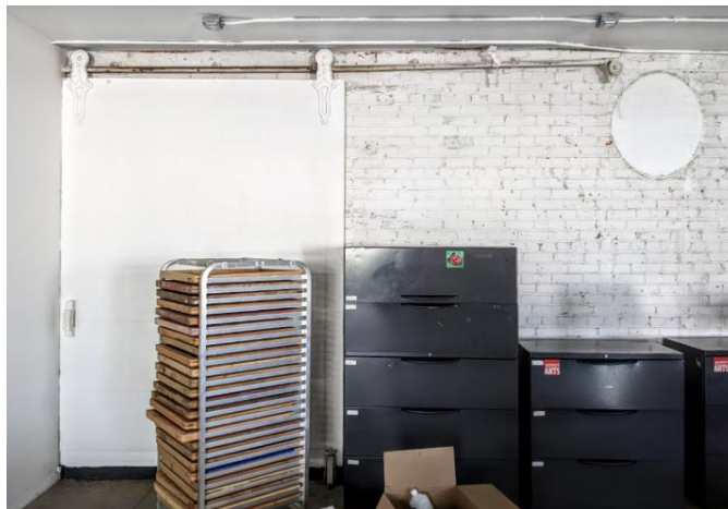
Figure 27. Door Hung on Round Track with Richard-Wilcox 542C Roller SOURCE: Sapphos Environmental, Inc., 2022
