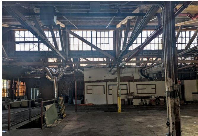
Figure 16B. Main Factory Space (facing north) SOURCE: Sapphos Environmental, Inc., 2022
