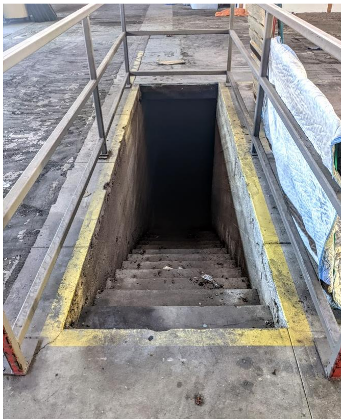
Figure 21. Basement Stairs, Main Factory Space SOURCE: Sapphos Environmental, Inc., 2022
