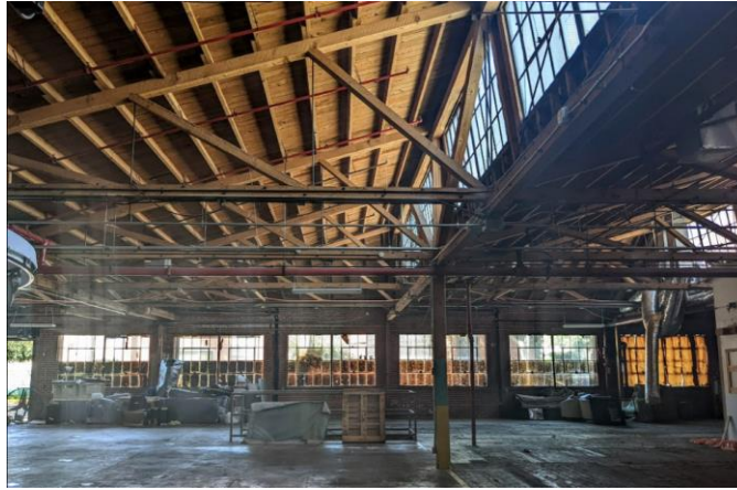
Figure 16A. Main Factory Space (facing west) SOURCE: Sapphos Environmental, Inc., 2022
