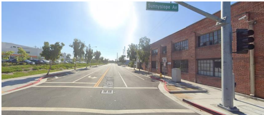
Figure 3B. Setting, E. Walnut Street (view facing east)
