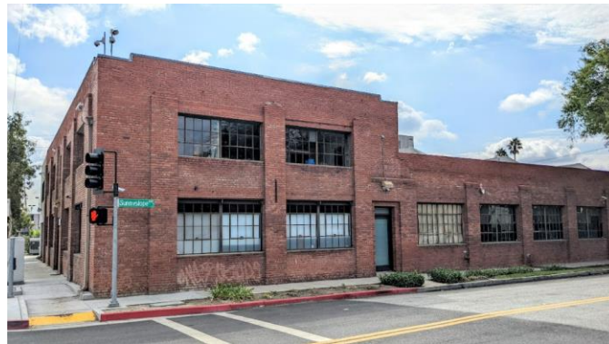
Figure 13. Northern and Western Façades (view facing southeast) SOURCE: Sapphos Environmental, Inc., 2022
