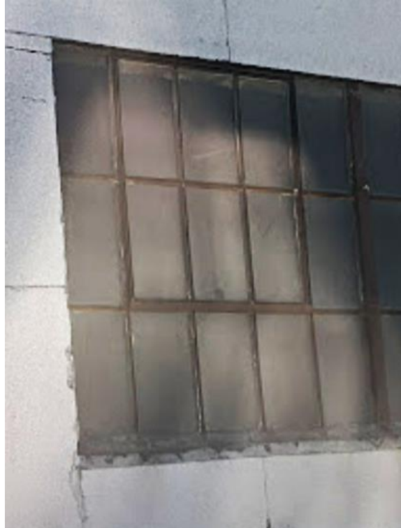
Figure 18. Detail of Mid-Sash Pivot Window (facing south from second-floor offices) SOURCE: Sapphos Environmental, Inc., 2022
