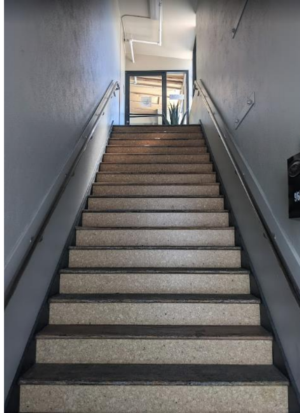
Figure 30. Staircase (leading from west entrance to second floor) SOURCE: Sapphos Environmental, Inc., 2022
